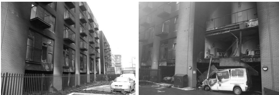
Figure 3 & 4 – example of the hazards of ventilation openings adjacent to a buildings facade
