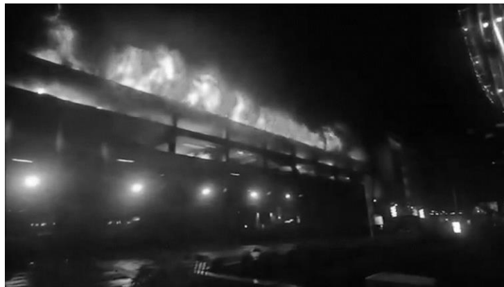
Figure 2 - Fire spread between floors via ventilation openings.
