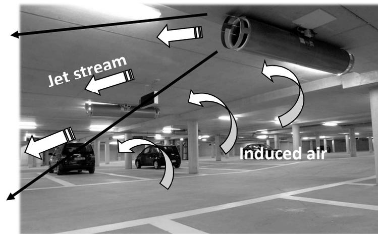
**FIGURE 9** – Diagram showing principle of induction of airflow
