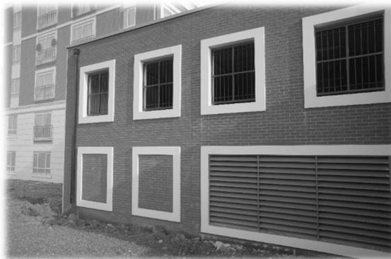
**FIGURE 4** – ASG “Low loss” louvre at the discharge of a car park extract chamber
